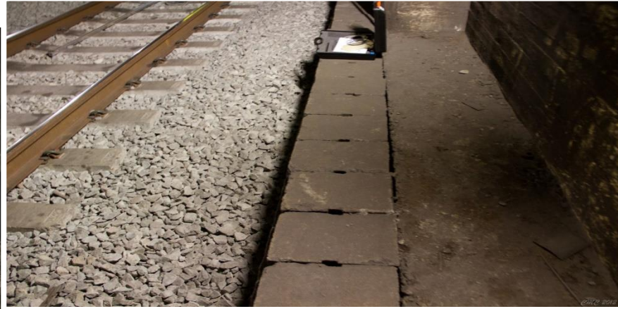
SITUATION BEFORE THE PROJECT : escape routes and cable duct
