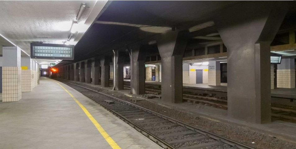
SITUATION BEFORE THE PROJECT Open structure
